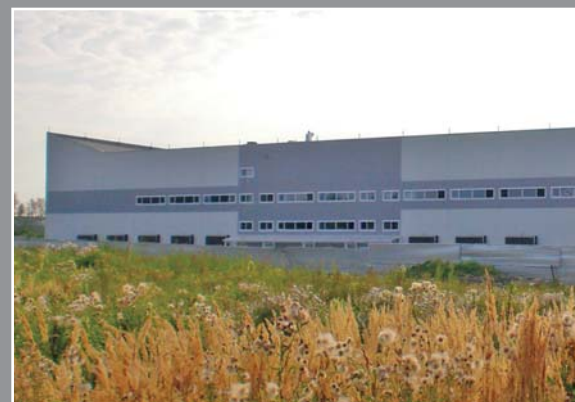
Delivery of sandwich panels, more than 12,000 m 2
