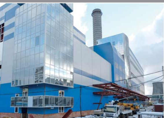
Construction and assembly operations, Delivery of sandwich panels 12,000 m 2
