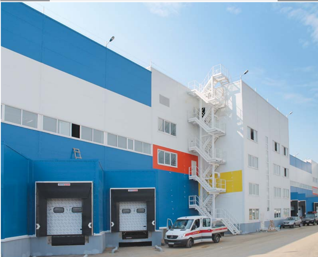
Planeta manufacturing and storage facility, Leshkovo village, Pavlo-Slobodskoe rural settlement, Istra district, Moscow region (2012-2013)
