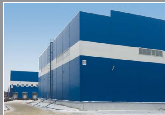
Delivery of sandwich panels, more than 100,000 m 2
