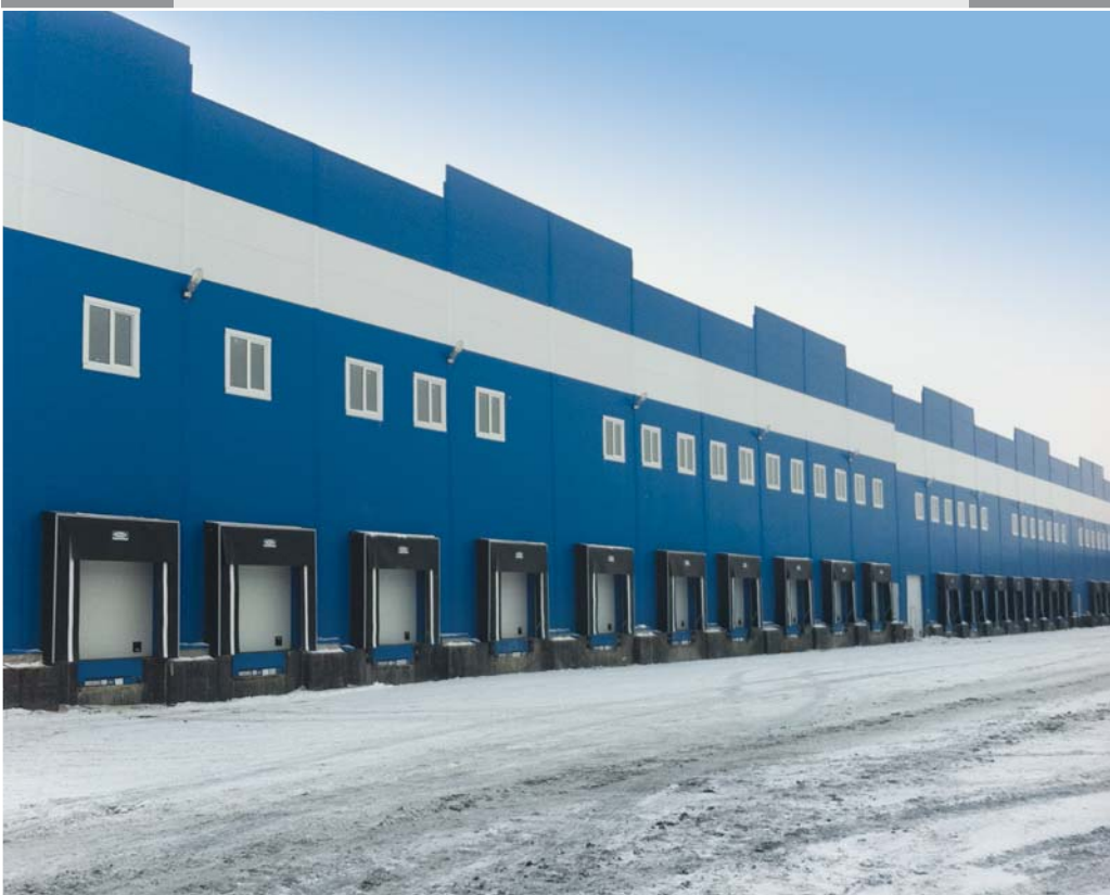
Atlant Park manufacturing and storage facility, Obukhovo urban-type settlement, Noginsk district, Moscow region (2011-2014)
