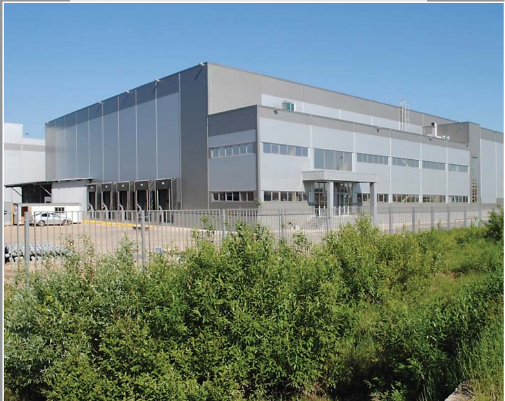
Dialog Invest office and warehousing facility, Leshkovo village, Moscow region (2012)
