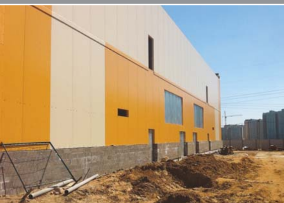
Construction and assembly operations, Delivery of sandwich panels 10,800 m 2
