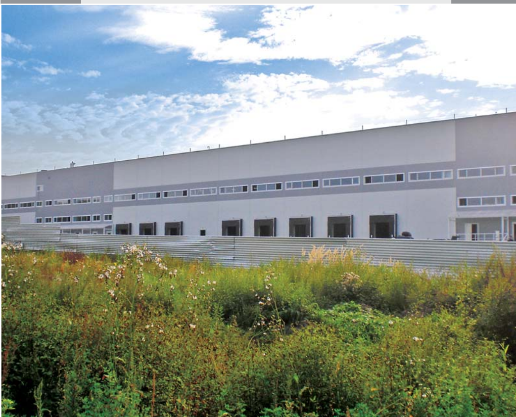
Logistics hub in the area of the Vostochny industrial park, Noginsk, (2013)
