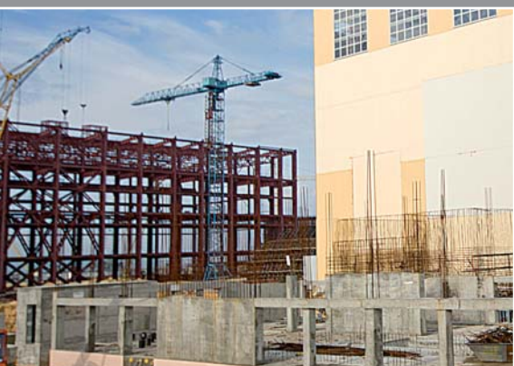
Metal structures 300 tons, Delivery of sandwich panels 20,000 m 2
