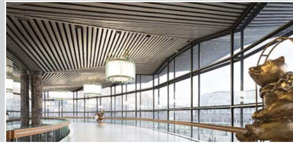
Capital repairs of the administrative and actors' modules (stylobate) total area 10,500 sq.m The work is performed within the framework of the program of the Ministry of Culture of the RF.
