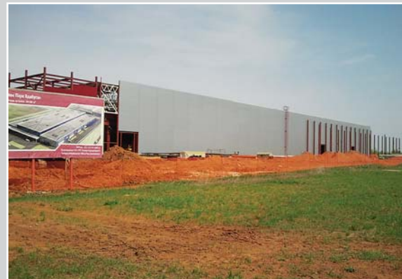
Supply of sandwich panels 14,000 sq.m
